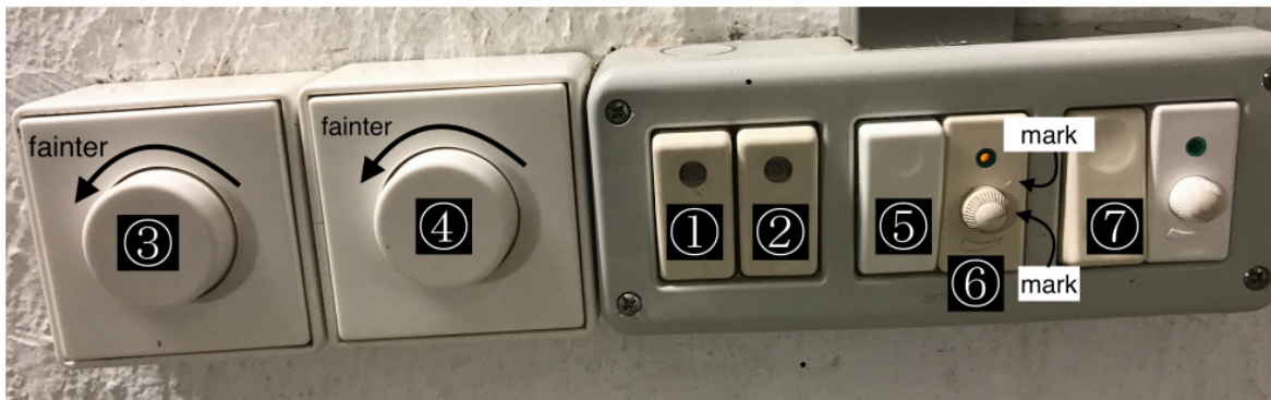
Figure 2: The dome light switches on the TCS dome.
